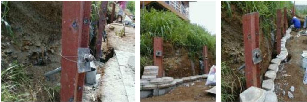
Soil Nail seen inserted through I Beam Post, First course of LocBlocs laid on CHB course laid in front of I-Beam
