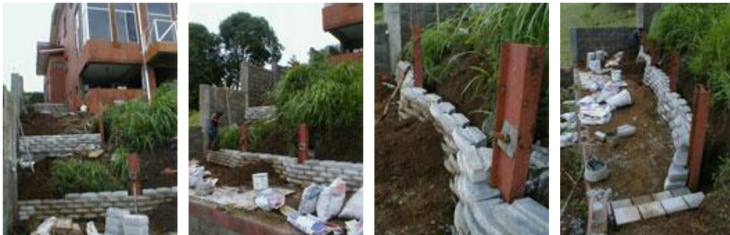
Soil Nail seen inserted through I Beam Post, First course of LocBlocs laid on CHB course laid in front of I-Beam
